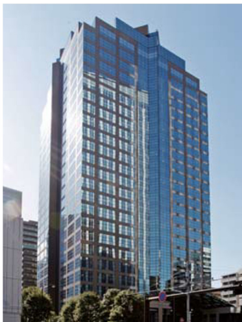
Nishi-Shinjuku Mitsui Building
